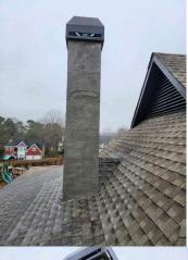
Applied mortar to the new chimney structure, we allowed 48 hours or cure time due to the lower temperatures outside prior to applying the new stone finish.
