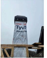
Installed the existing chimney cap, verified chimney was level and plum. Installed temporary support and bracing to ensure the chimney stayed level through the masonry process.
