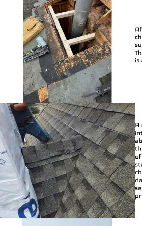
After demo of the existing wood rot chimney, we went ahead and replaced the support block framing just inside the roof. This way the new chimneys entire structure is all new and secured as best as possible.
